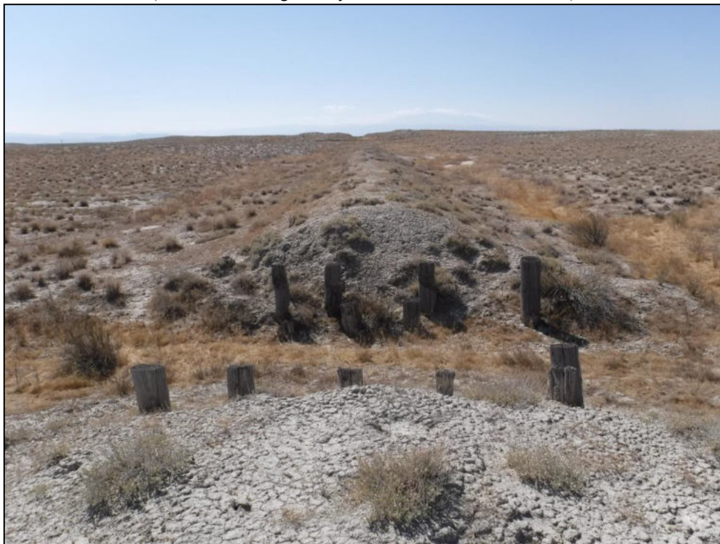
Figure 6. 42GR935 Feature 2, bridge remnants, view southwest (Roll 20-808, image 17, by Natasha Krasnow, 09/01/2020)
