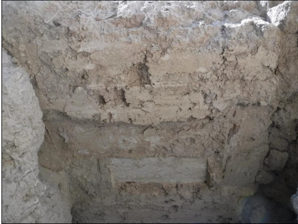
Figure 5. 42GR935 Feature 1, earthen bridge, detail of wood plank impression (Roll 20-808, image 08, by Natasha Krasnow, 09/01/2020)
