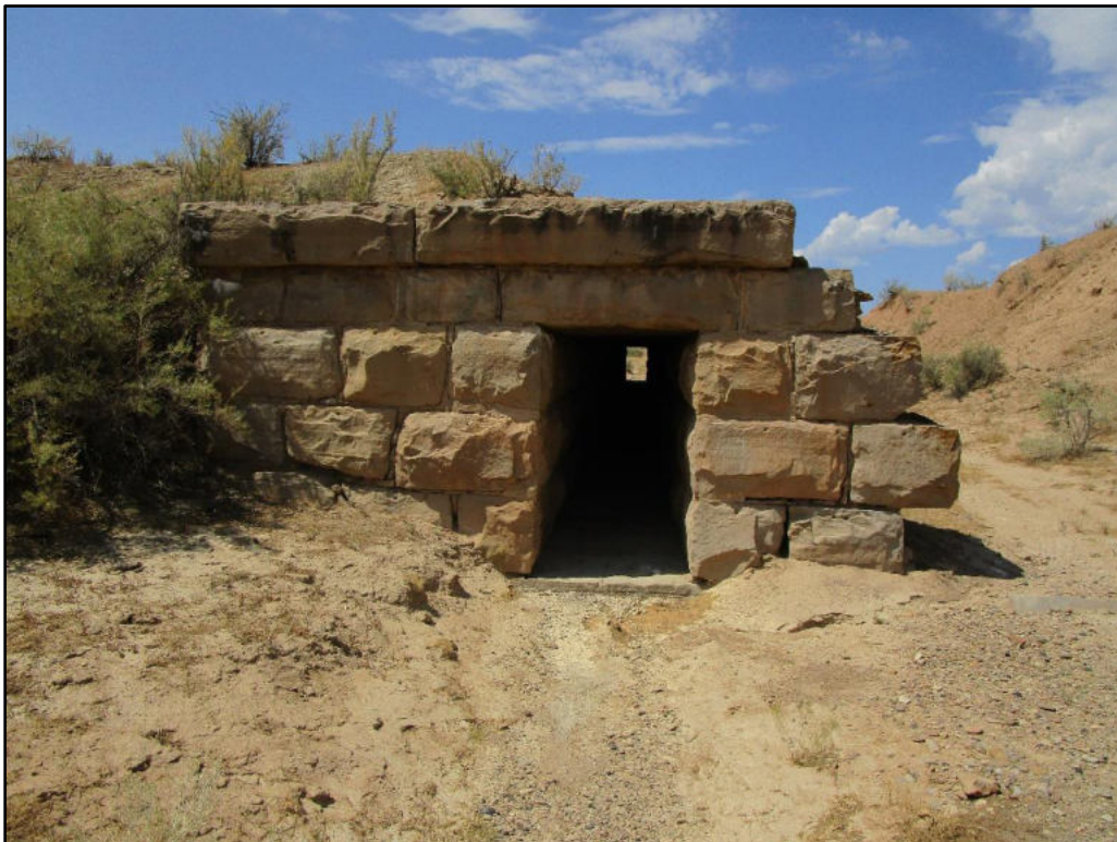
Site 42GR935. Site overview showing sandstone culvert visible outside of project area from survey line 12 at UTM 646221mE/4324017mN; view to the west.
