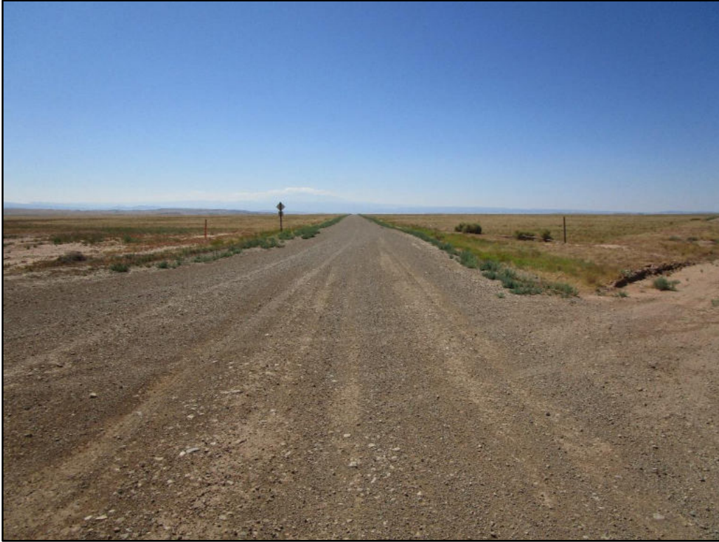
Site 42GR2305. Site overview from north end of segment at junction with Danish Flat Road (42GR7591); view to the south.
